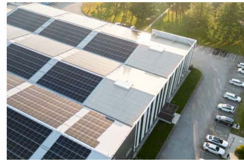
We have our own solar power plant and heat pump. Renewable energy source for electricity: 29% in 2022 | 72% in 2023 | 100% by 2024.
