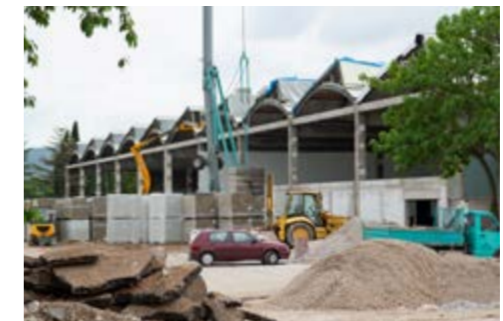
We breath new life in old degraded buildings. We reuse a lot of the construction materials from the demolition work.
