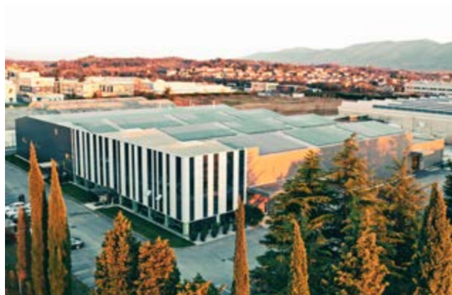
Solar panels generate enough energy to run the factory and HQ autonomously.
